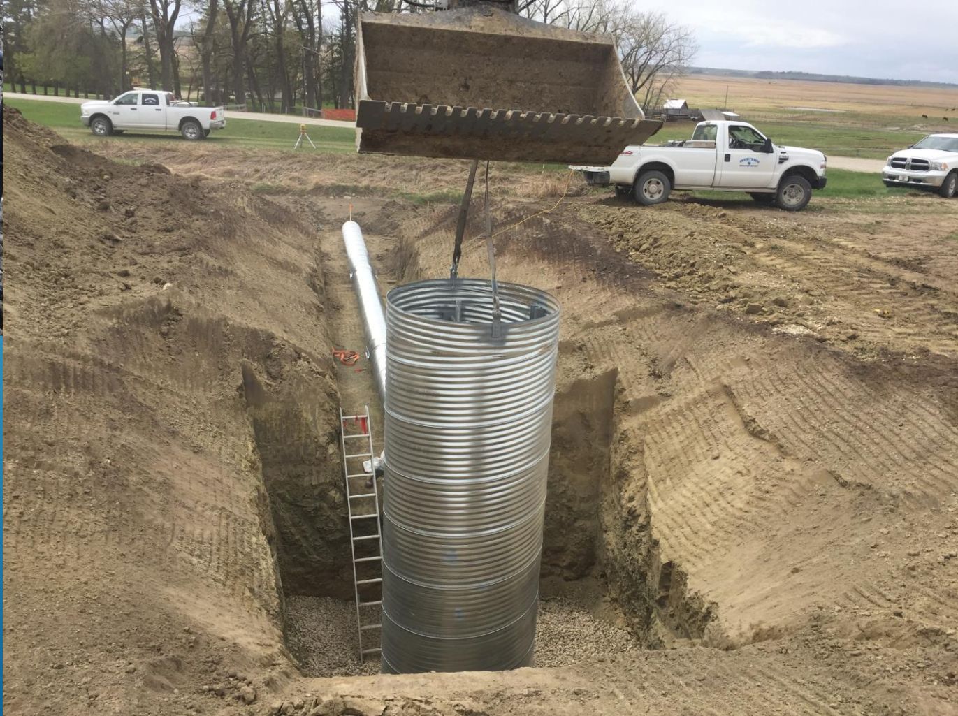
Irrigation standpipe and inlet installation for turbine pump
