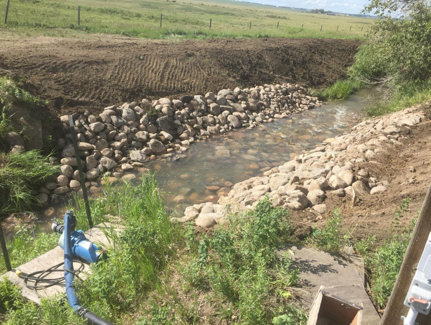
Washed out drop pipe replaced with rip rap
