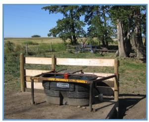
The water storage assistance program that the WID offers can help out with more than just digging a hole. We can also help with installation of stock waterers that work off of pipeline pressure or solar pumps from dugouts. In both instances, water quality is improved for the livestock and less water can be diverted to service the same animals. Everyone makes a positive gain, the producer, the animal and the District.
